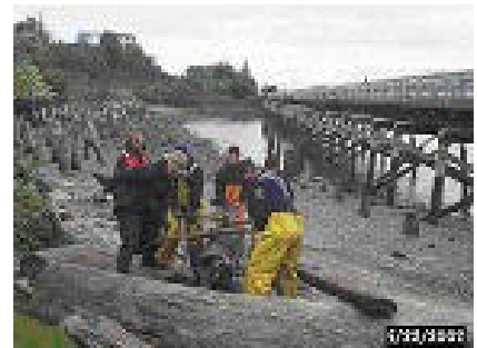
Creosote log removal project.
